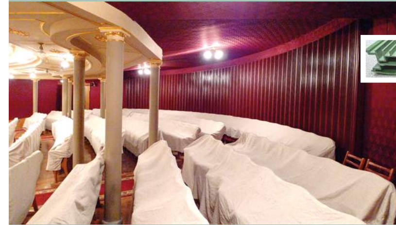
Diffusion-sound-absorbing panels in the Lviv National Opera
